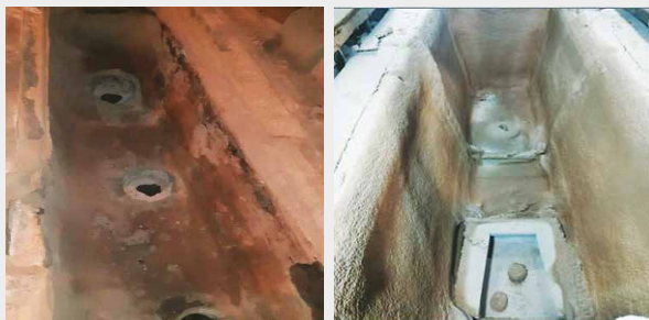
Tundish after installation
